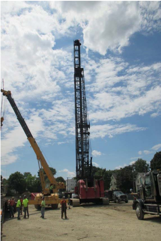
Installation of Foundations
