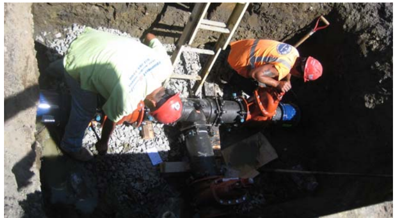
Utility Tie-Ins in Street
