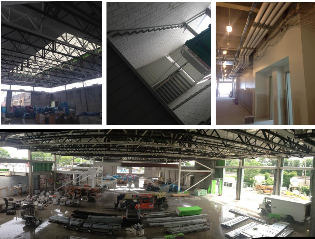
Status of Interior Construction
