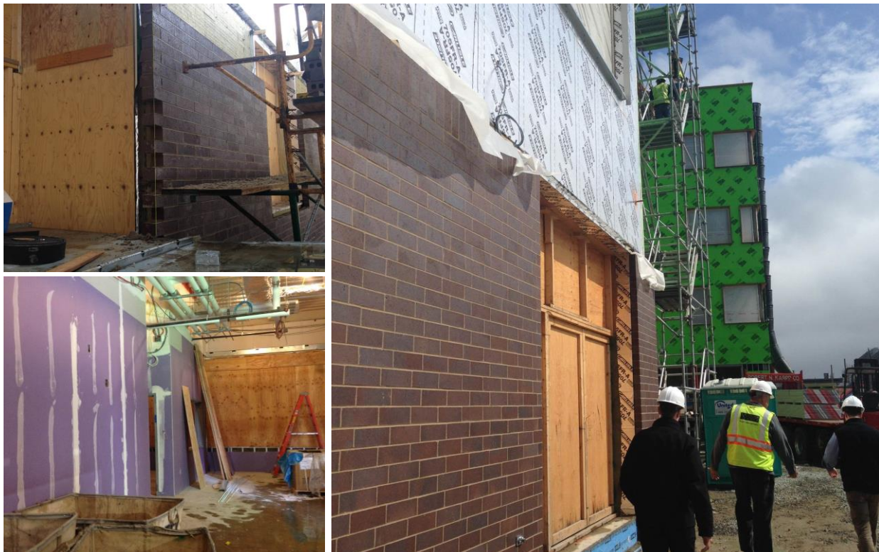
Status of Exterior and Interior Construction
